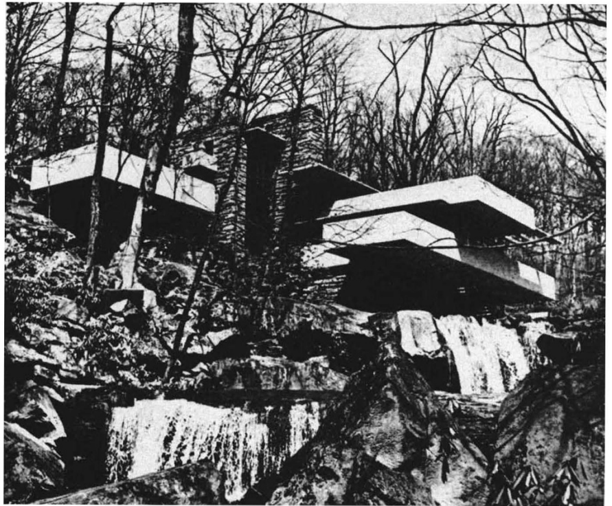
A house designed by Frank Lloyd Wright and built in Pennsylvania in 1935. This illustration, from the second edition of American Buildings , by James Marston Fitch (Houghton Mifflin, Boston, 1972; $15.00), “tells us nothing about conditions inside where cascade is invisible, perceivable as noise, humidity chill”.
